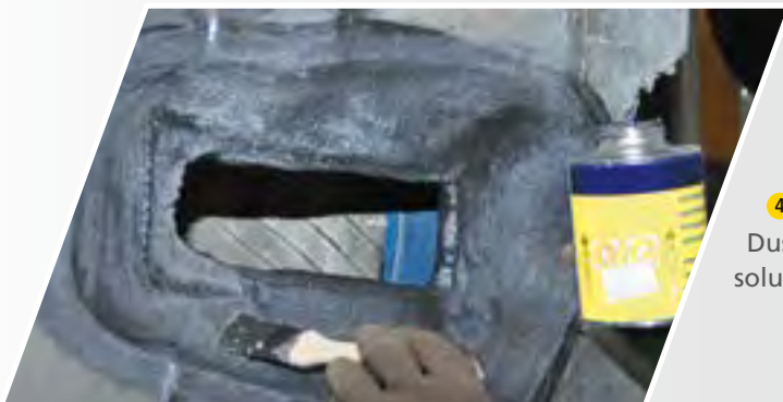
Application of rubber solution
