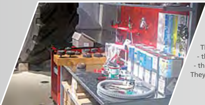
Preparation of the repair products
