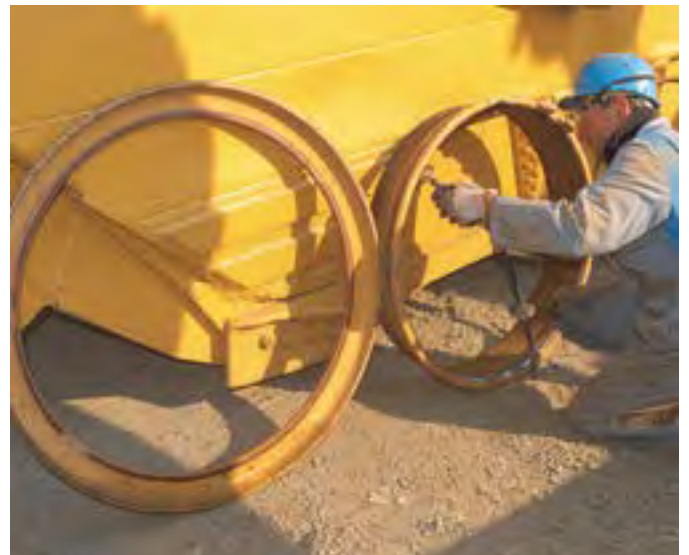
Cleaning and repainting the rusty areas of metal parts
