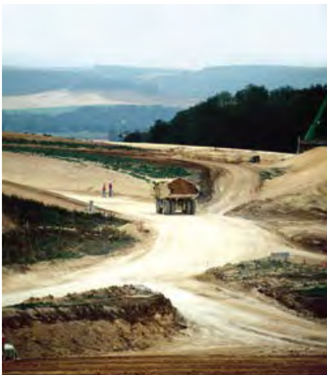
Appropriate design of site roads reduces tapered wear
