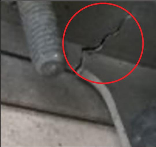
Figure 2. Example of head unit cracking along radius
