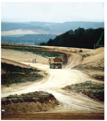
Appropriate design of site roads reduces tapered wear
