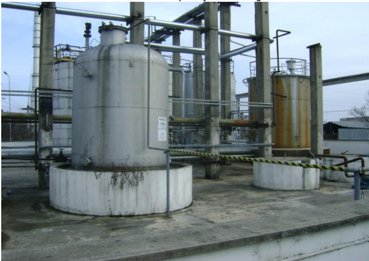
Zona stocare plastifianti – rezervor solvent EXXSOL™ DSP 100/160 – imagine 2
