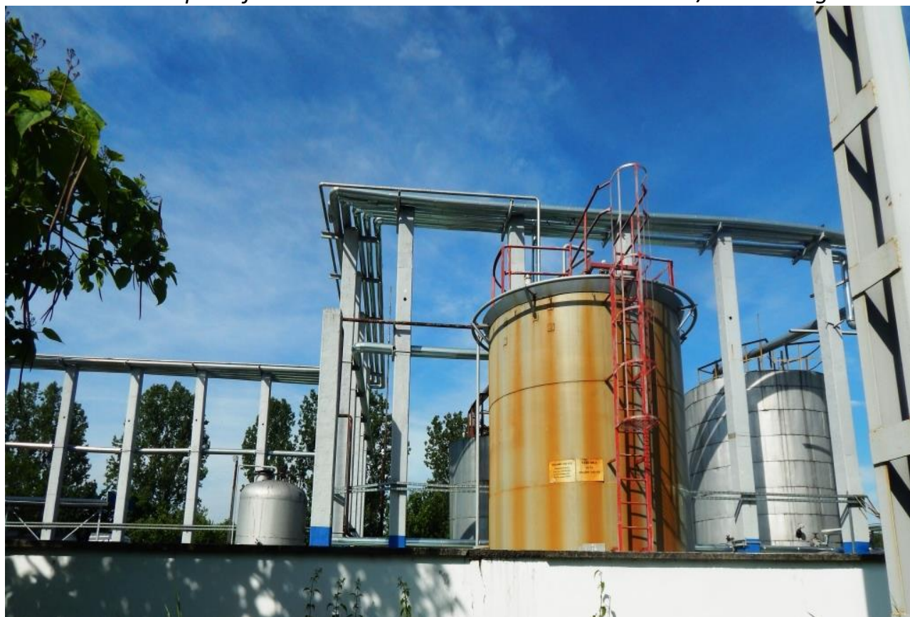
Zona stocare plastifianti – rezervor solvent EXXSOL™ DSP 100/160 – imagine 2
